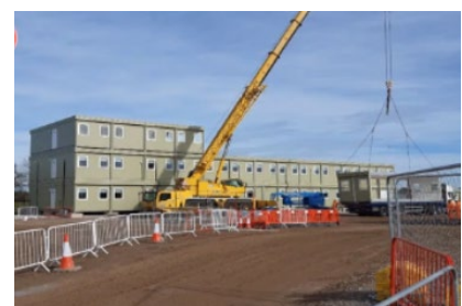
West Street compound set-up
